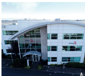
Westland House, Dublin 12
